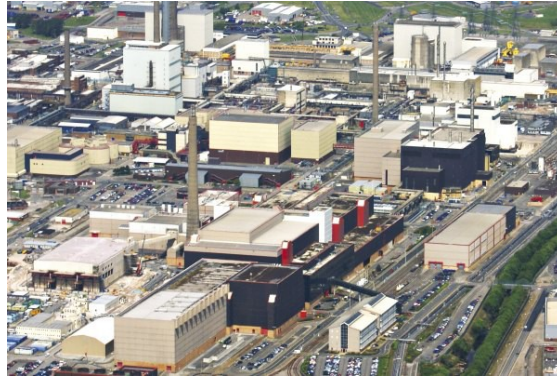
The Thermal Oxide Reprocessing Plant (THORP) at Sellafield, UK The smaller black building to the rear is the vitrification plant. (Sellafield Ltd.)
