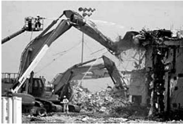
FIGURE 14.10 Typical large equipment demo.
