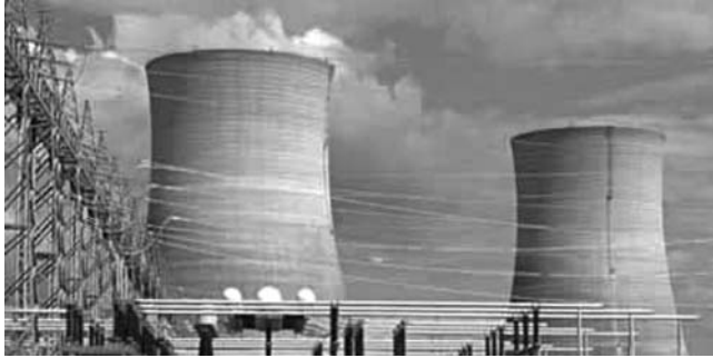
FIGURE 14.7 The Tennessee Valley Authority's Sequoyah nuclear power plant.
