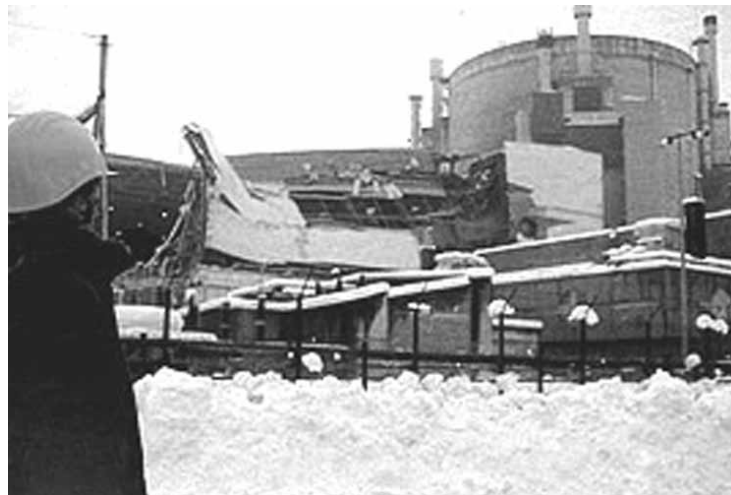
Figure 2.5 Superphénix collapsed turbine hall roof. Photo: Dissident-Media.
