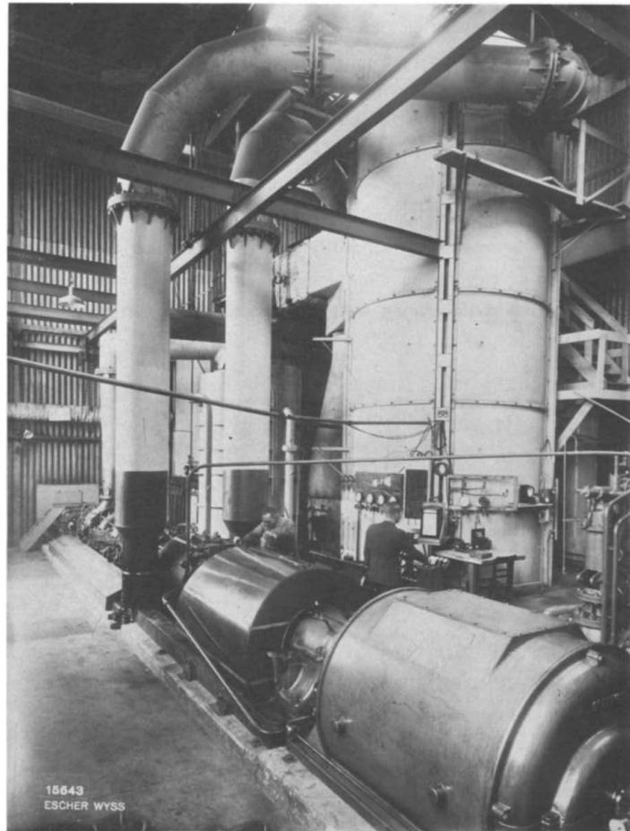
**Figure 8** The Escher Wyss AK-36 test plant [20]
