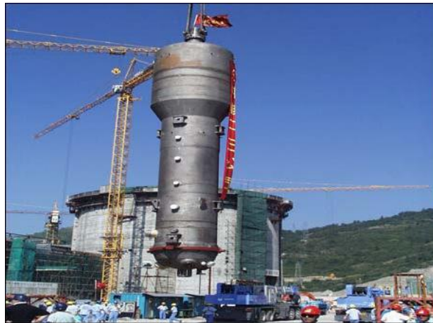
Figure 19. Installing a steam generator at Qinshan 3-1 in China using the open top installation method.
