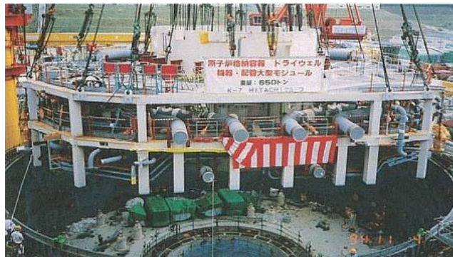
Figure 20. Installing the upper drywell super large scale module at Kashiwazaki Kariwa-7 in Japan.
