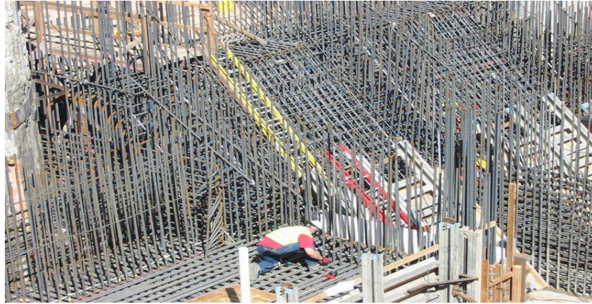
Figure 21. Steel plate reinforced concrete and slip-forming.
