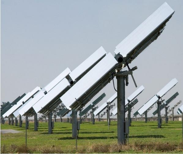
**Figure 1.12** Photo of fifth in the world 1.2-MW<sub>el</sub> concentrated photovoltaic (PV) solar power plant (Spain). The plant has 154 two-axis tracking units, consisting of 36 PV modules each, which cover an area of 295,000 m<sup>2</sup> with a total PV surface area of 5913 m<sup>2</sup>. The plant generates 2.1 GWh each year, and the conversion efficiency is 12%.
